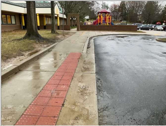
ACCESSIBLE ROUTE TO PLAYGROUND
