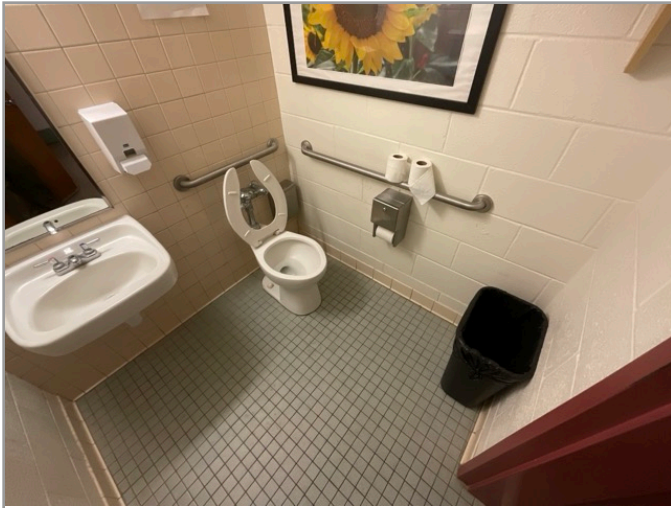
TOILET STALL OVERVIEW
