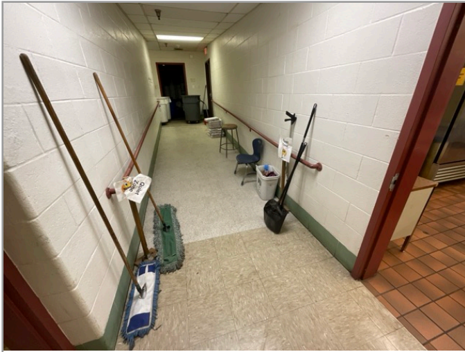
ACCESSIBLE INTERIOR RAMP
